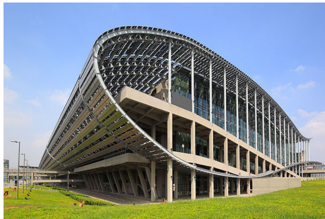
Figure: Amazing steel structure (from clsteel)
