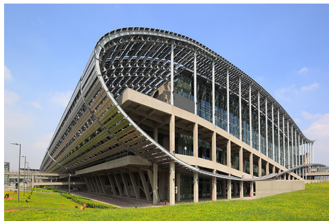
Figure: Amazing steel structure (from clsteel)
